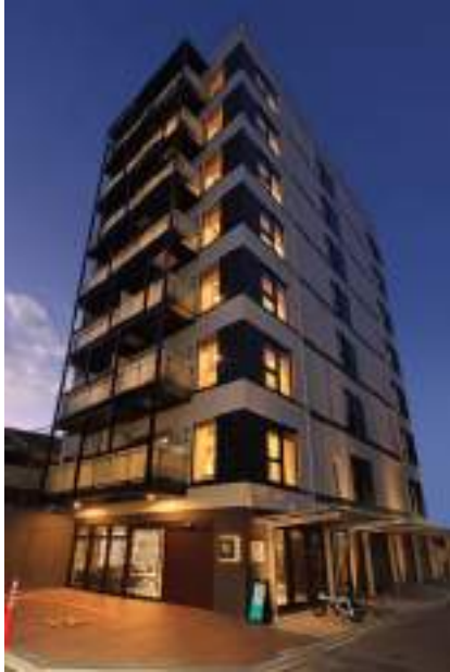
13_CAPS7847_外観南東面(夜景)_修整2
