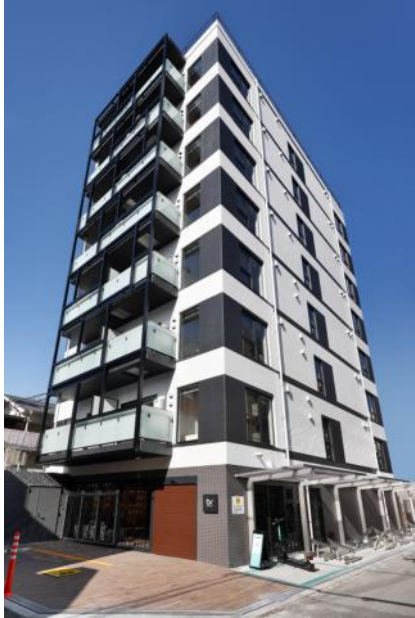
01_CAPS7444_外観南東面_修整2
